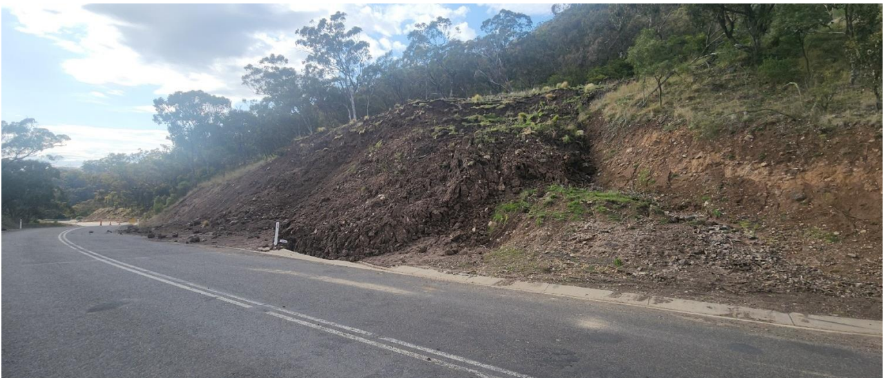
Figure 2 View of slope failure on Merriwa Road (photograph taken on 8 September 2025)
